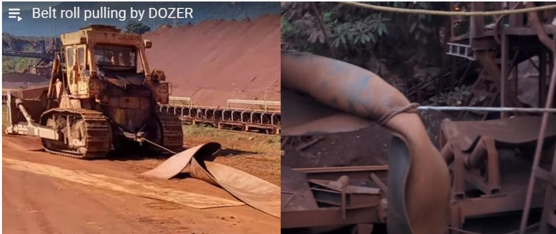
Figure 17 - Lashing of the belt
