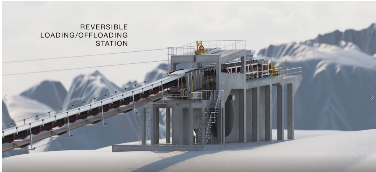
Figure 2 – Reversible loading / offloading station
