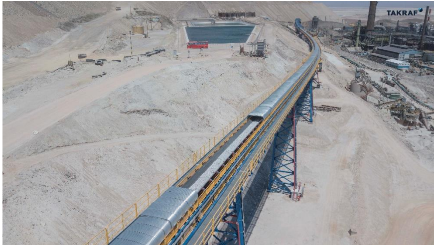
Figure 12: Overland conveyor OLC-01 passing over existing infrastructure.
