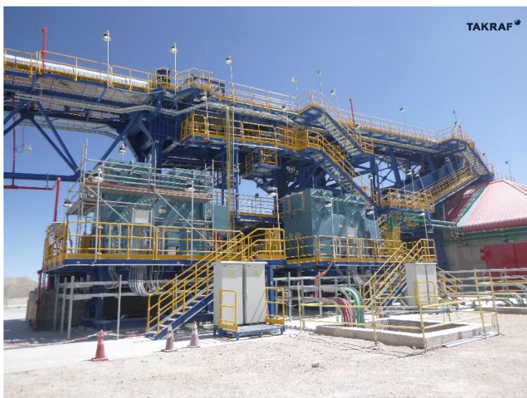
Figure 13: Bunker building with material discharge from the overland conveyor OLC-01.
