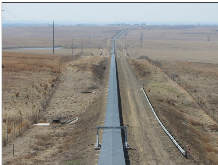
Figure 2: Impumelelo overland conveyor
