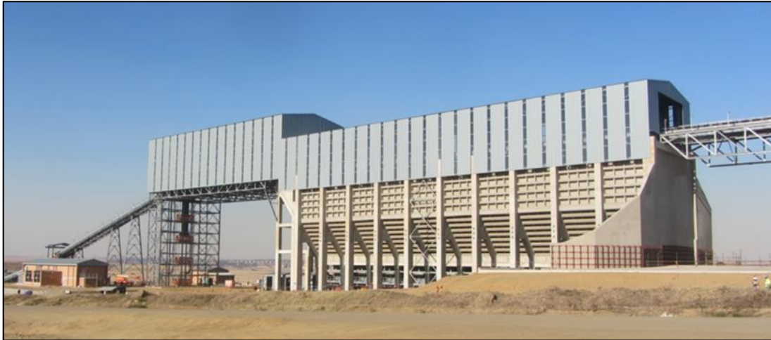
Figure 7: Shondoni 15000 ton bunker
