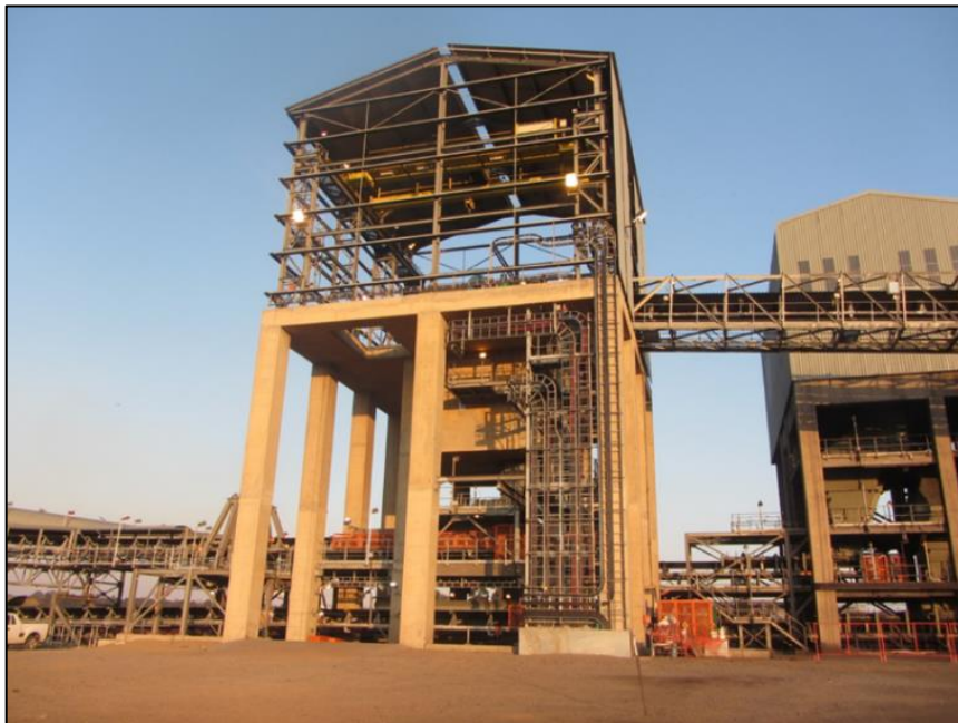
Figure 14: Head end with bin (during construction phase).
