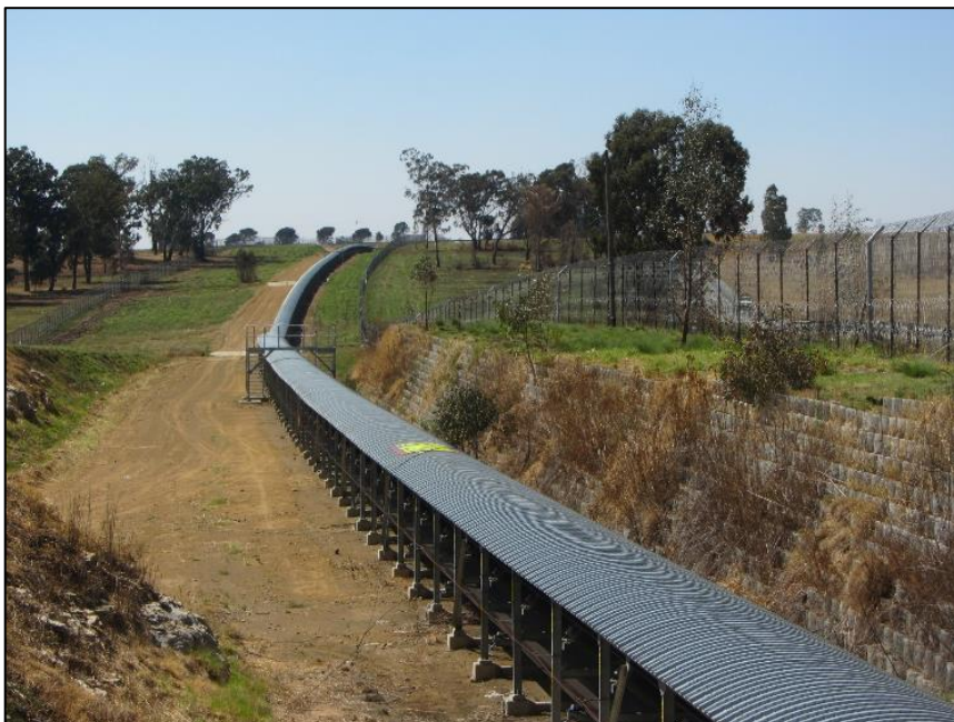
Figure 12: Shondoni overland conveyor
