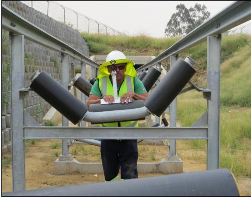
Figure 13: Alignment of idler frames.
