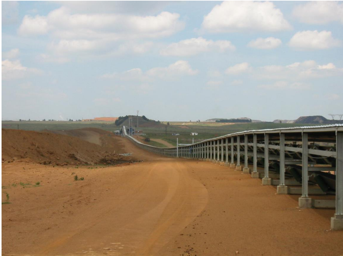
Figure 9. Overland conveyor KW-05 looking towards the head of the conveyor.
