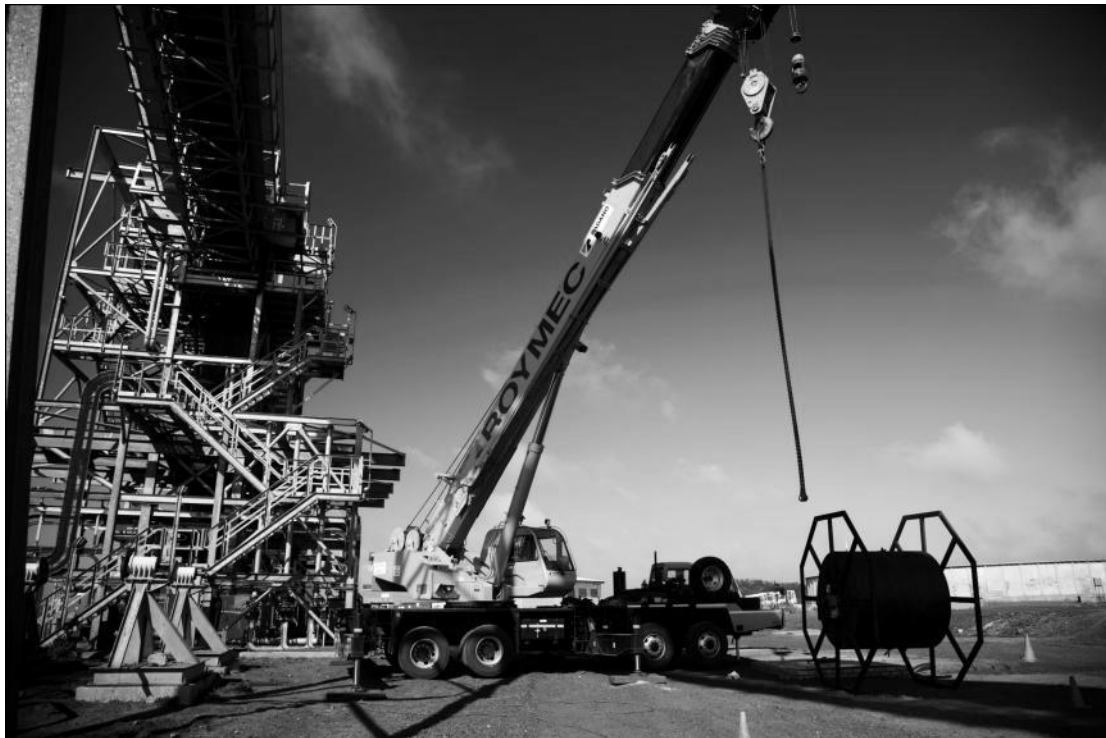
Figure 7. Belt installation
