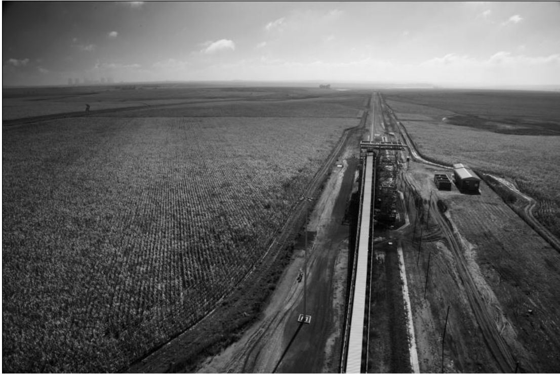
Figure 1. Crushing and screening plant
