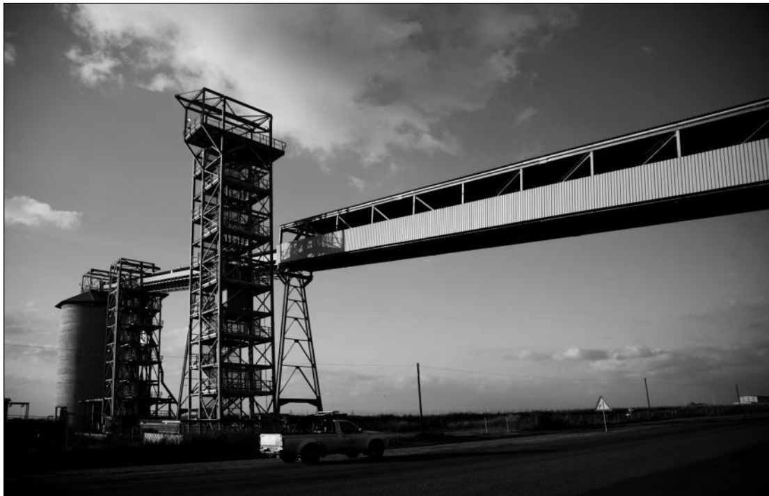
Figure 6. Gantry spanning public road
