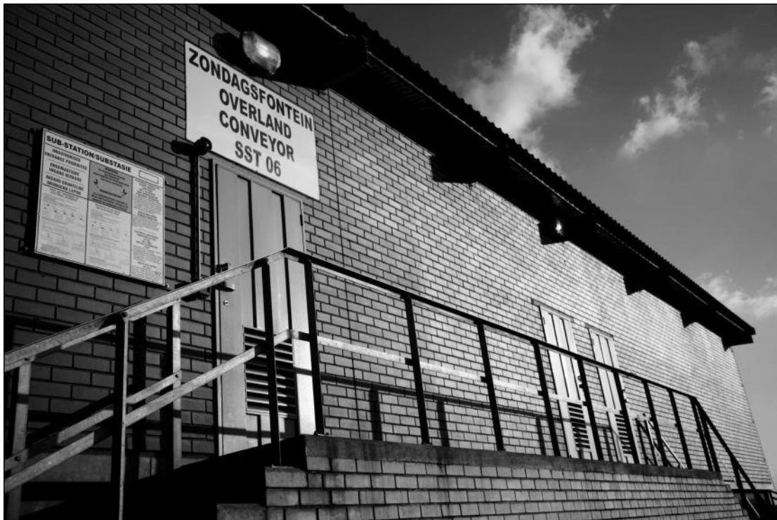
Figure 8. Sub-station at the head end
